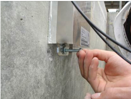
Fig. 2.5 Applying the washers and hexagon nuts
