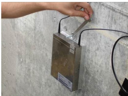
Fig. 2.12 Fastening hexagon nuts
