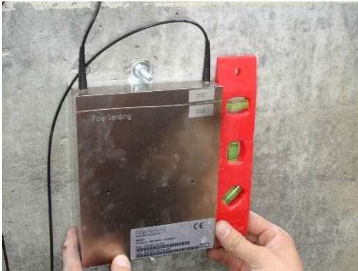
Fig. 2.6 Vertical alignment using a bubble level
