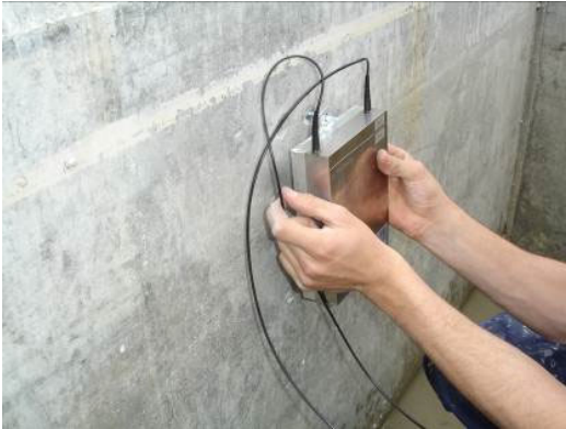
Fig. 2.4 Placing the sensor on the supports
