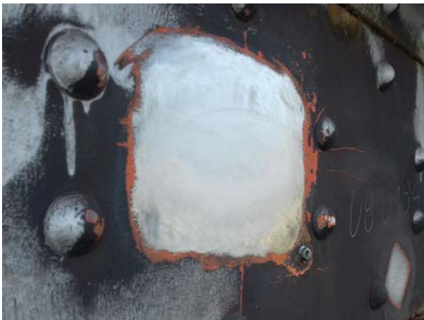
Fig. 2.5 Ready to weld surface
