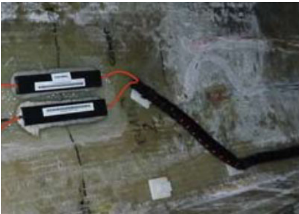
Fig. 2.36 Cable protected with corrugated tubes
