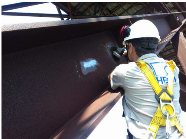
Fig. 2.2 Surface deburring
