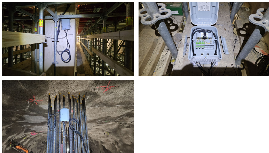
Fig. 2.11 Protection box for optical connections protection examples
