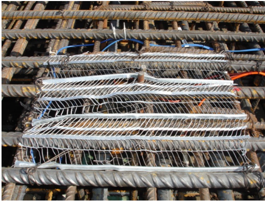
Fig. 2.18 Sensor area protection
