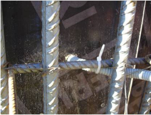
Fig. 2.9 Direct exiting from the formwork (inside view)
