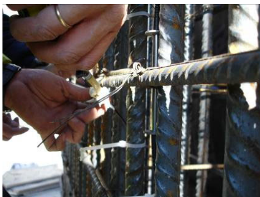
Fig. 2.16 Protection tube sealing
