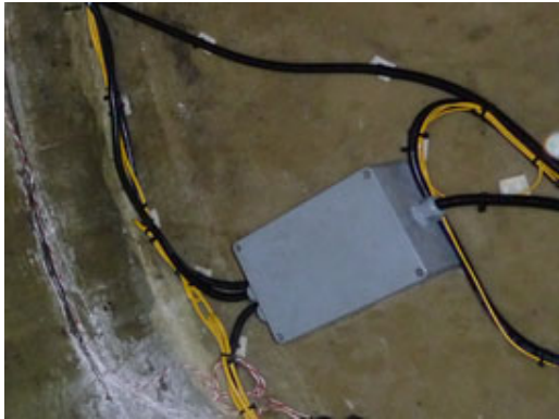
Fig. 2.32 Protection boxes for extra cable and connections
