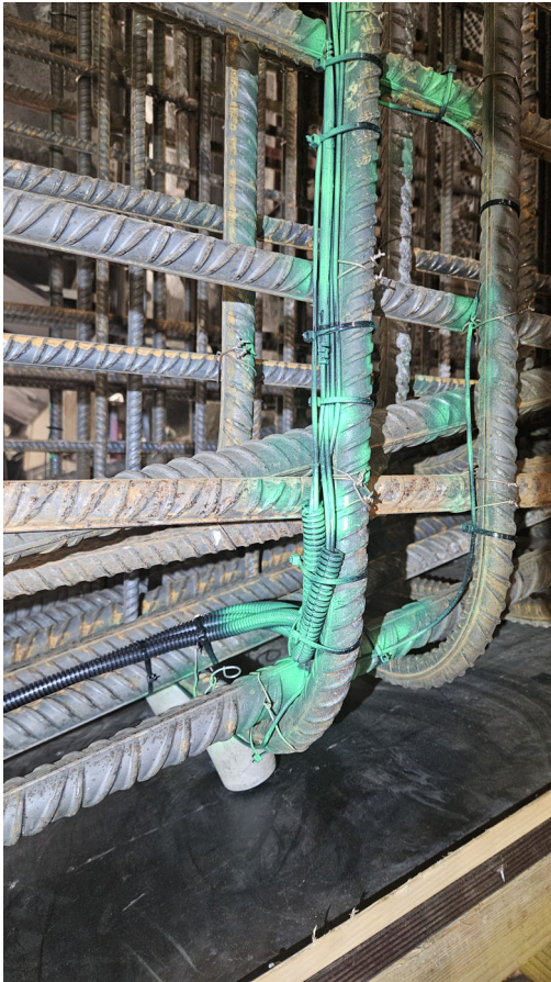
Fig. 2.8 Highlighted protection tube on delicate areas
