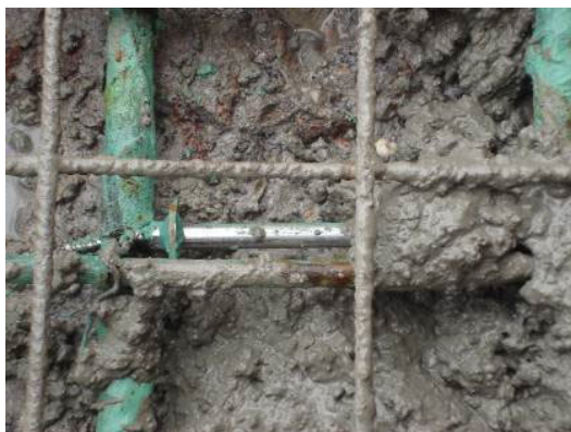
Fig. 2.17 Sensor during concreting
