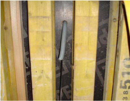
Fig. 2.10 Direct exiting from the formwork (outside view)
