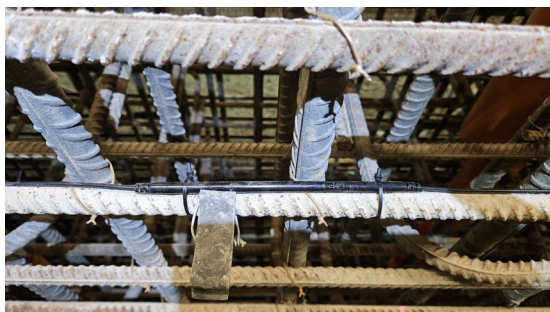
Fig. 2.15 Splice fixation
