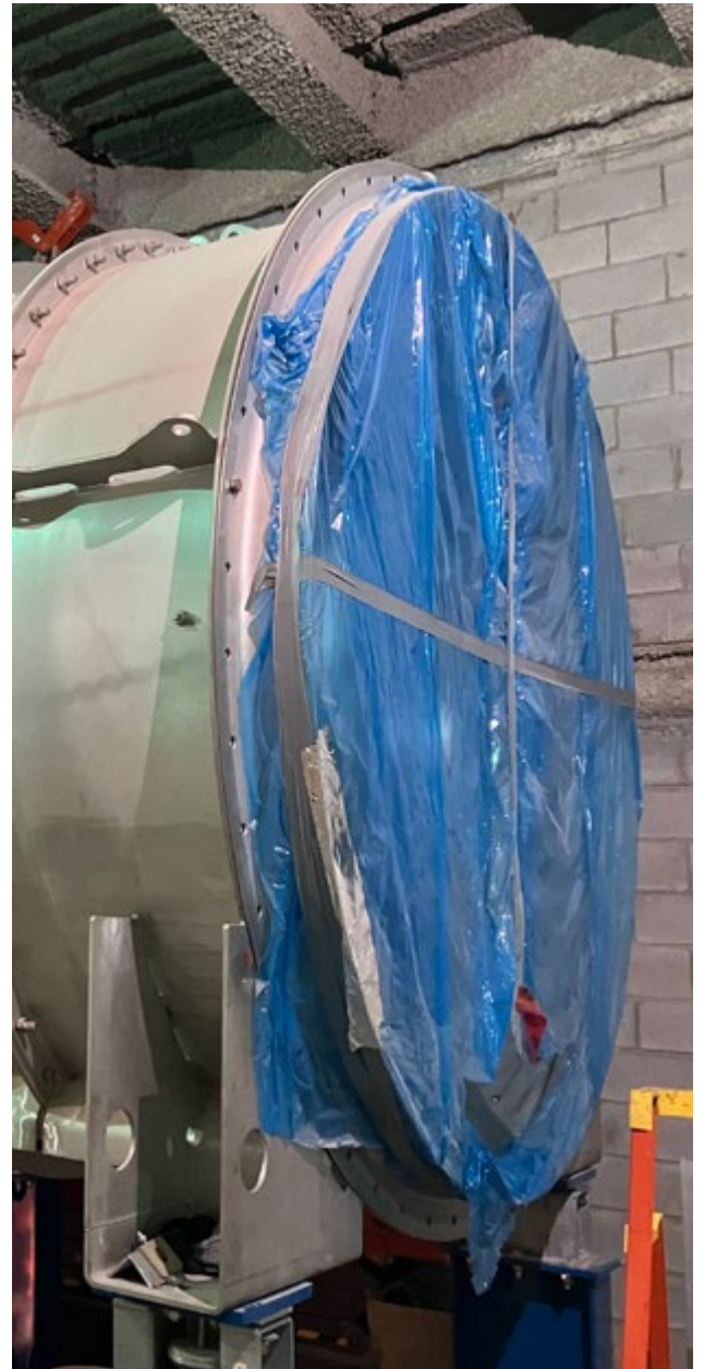
Fans used to aerate train stations
